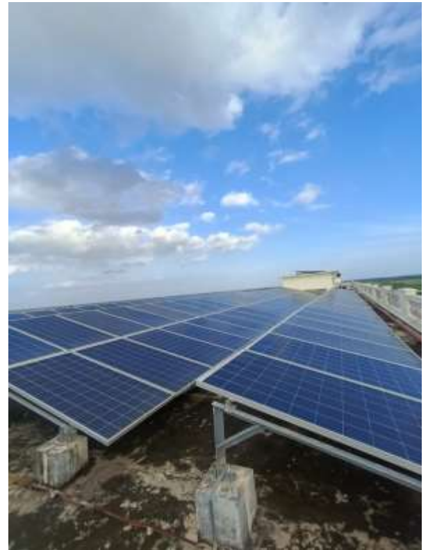
Fig.: 2.1- Solar Plant Installation on College rooftop
